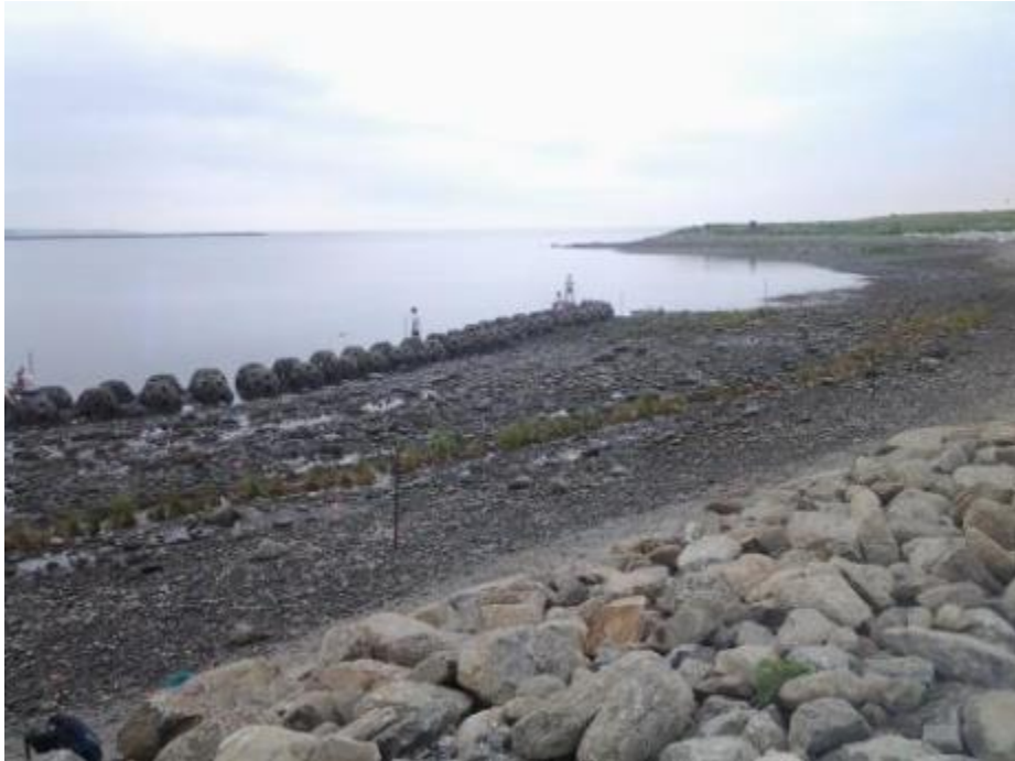
The living shoreline pilot project consisted of an artificial reef and intertidal marsh. This photograph was taken approximately three months after construction in July 2014. Note the gravel / cobble substrate.
