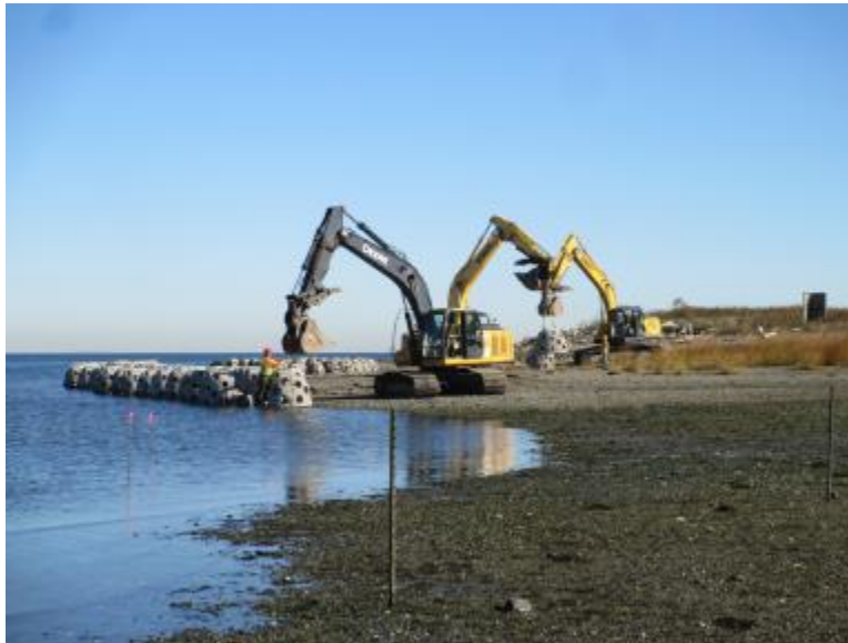
The artificial reef was constructed in five days between November 14 and 18, 2016. Construction occurred during low tide to minimize disturbance.
