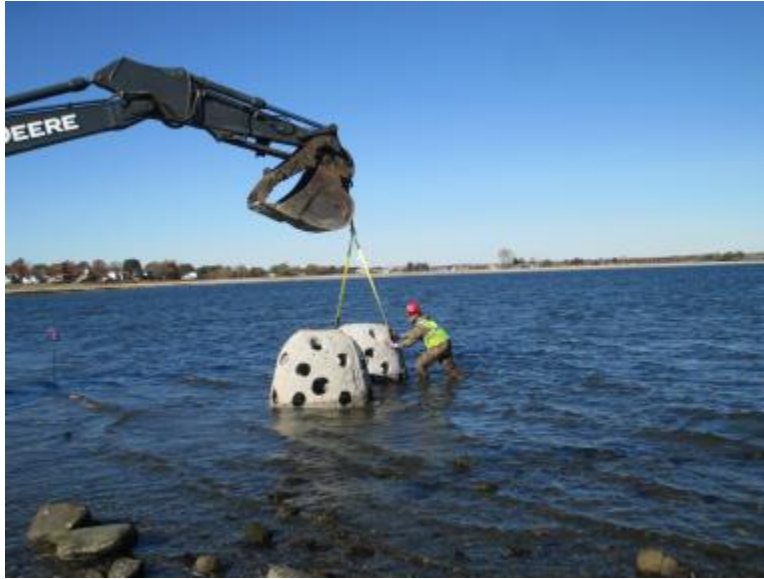
The first phase of the project consisted of expanding the artificial reef included in the pilot project. The reef was again constructed with precast concrete reef balls, which CIRCA match funds were used to purchase.
