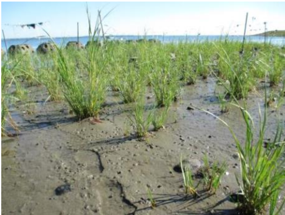
This photograph was taken approximately one and half years after construction in September 2015. The gravel / cobble substrate that was present prior to, and immediately following, construction has been covered / buried with fine-grained sediment. Over the three year monitoring period, up to 60 cm of sediment has been deposited in the project area. Intertidal marsh vegetation has become established and is beginning to thrive.
