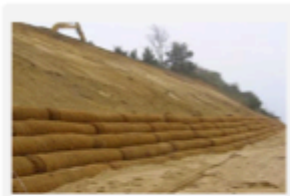
Bank Stabilization with Coir Logs. Photo courtesy of Wilkinson Ecological Design, Inc.
