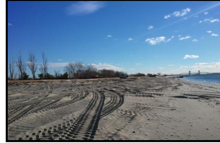
Plumb Beach: 155,000 CY
