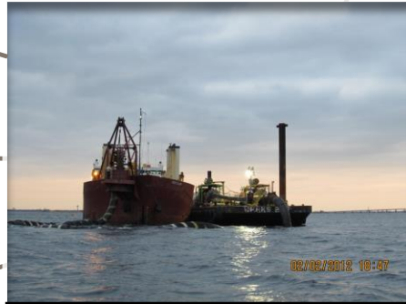
Harbor Deepening Project: ~50 M CY
