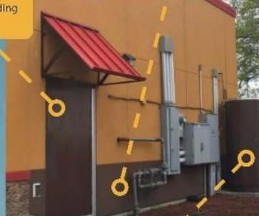
The "Elevation" of this new restaurant and its critical infrastructure were constructed above flood elevations, while maintaining ADA access from parking areas.
