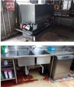
Figure 6. New London Fire HQ & EOC, Interior. First floor elevation and utilities 4 ft below BFE (behind flood wall). Recommended for floodproofing.
