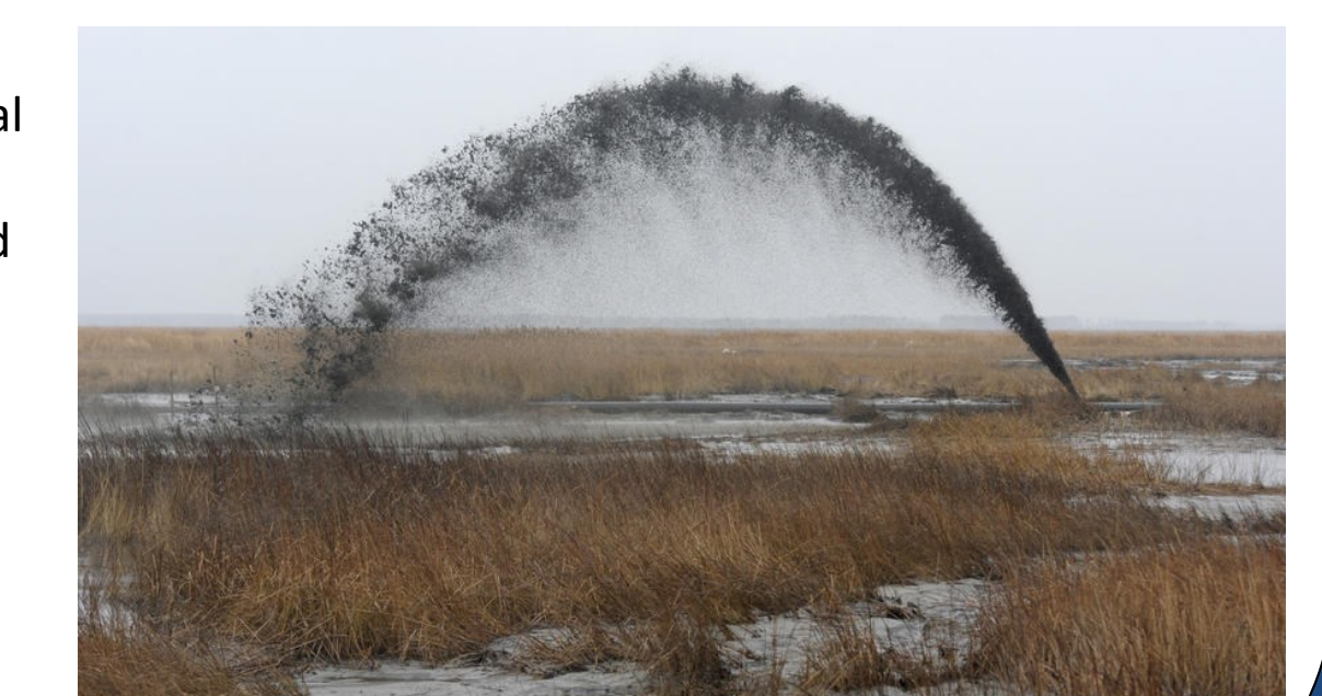
Blackwater National Wildlife Refuge - Dredge America
