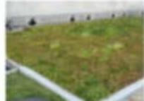
As a part of the Green Capital Project, a green roof was installed at the Connecticut State. The area consists of vegetated modular trays that include a growing medium planted over a waterproof membrane.
