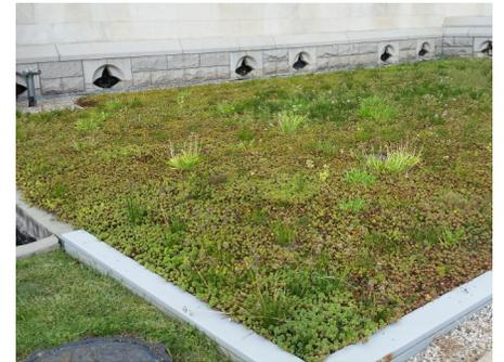
As a part of the Green Capitols Project, a green roof was installed at the Connecticut State. The area consists of vegetated modular trays that include a growing medium planted over a waterproof membrane.
