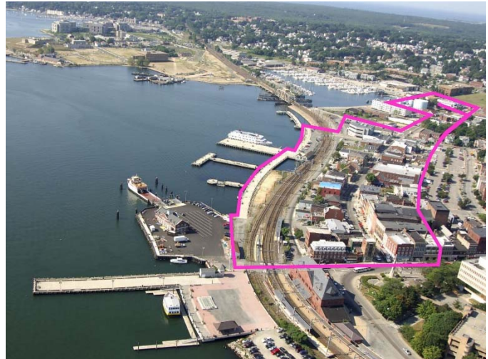
South Water Street is on the edge of the Thames River. The area is historically vulnerable to flooding due to its low-lying
