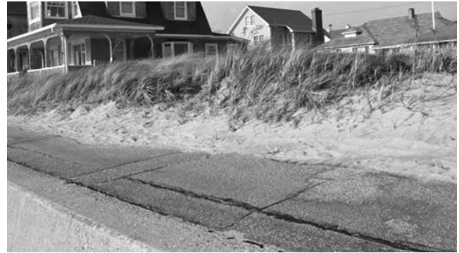
Figure 3. Even on very small sites with less than ideal conditions, beach grass can trap windblown sand, creating a protective barrier to the structure landward. Beach grass was planted on a 6-m-wide property located above a 1-m-high seawall, topped by a paved sidewalk. The trapped sediment is now over 1 m high, and the beach grass is colonizing neighboring properties.
