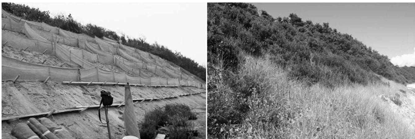
Figure 1. Erosion of a soft bluff can be mitigated by regrading the bank to a stable slope and then planting it with appropriate vegetation to provide a stabilizing root system. This project used a baffled cell technique and biodegradable matting to provide protection while the native plants became established. Temporary scaffolding was erected to reduce soil compaction and erosion during the construction phase. The mature native plants withstood Hurricanes Irene and Sandy with no major erosion, bank sloughing, or plant loss (New England Environmental, Inc., 2015; photo credit: New England Environmental, Inc.).
