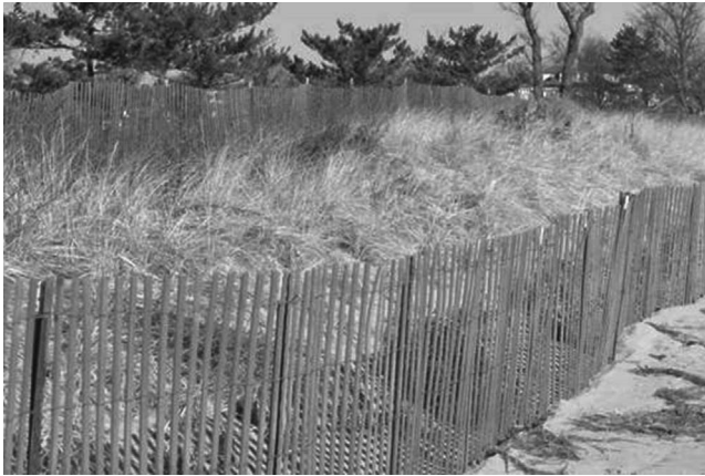
Figure 2. A sand dune is recreated where the nature dune existed before being destroyed during Hurricane Sandy. The dune has been planted with native vegetation. Sand fencing aids natural dune formation while protecting it from damage by foot traffic.
