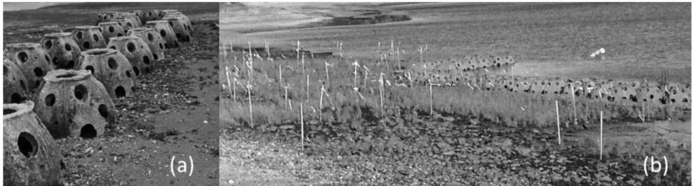
Figure 8. Wave attenuation devices, such as reef balls, are designed to attenuate waves while providing benthic habitat. Reef balls are available in several sizes. The size selected is dependent on design water depth of the reef. Typically, the height and width of the reef is similar to the design parameters of a traditional breakwater. These reef balls are deployed off Stratford Point, Connecticut, to provide protection to a created fringe marsh (photo credit: (a) A. Dolan, Graduate Student, Sacred Heart University via J. Mattei, personal communication; (b) J. Mattei, Department of Biology, Sacred Heart University).
