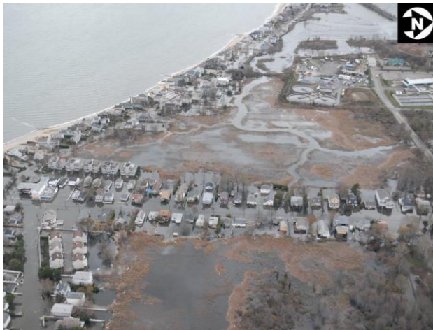
Figure 1-1 Flooding in Fairfield Beach after Hurricane Sandy
