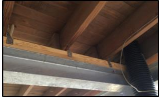
(b) Steel girders
