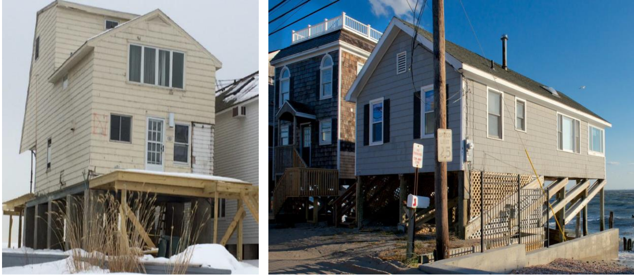
Figure 1-3 Elevated buildings in Fairfield after Sandy
