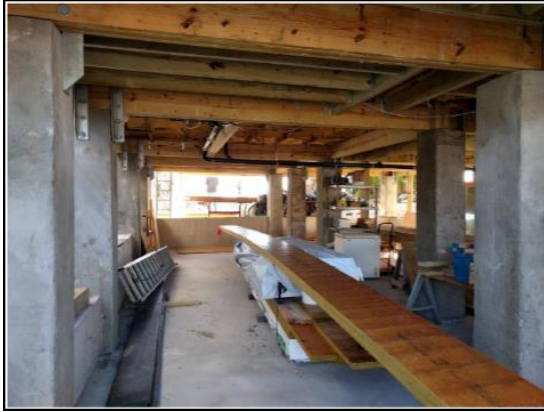
(a) Concrete piles
