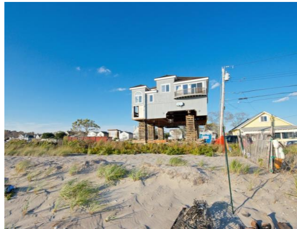
Figure 1-2 Elevated home on Fairfield Beach Road showing the overall response of neighborhood after Hurricane Sandy
