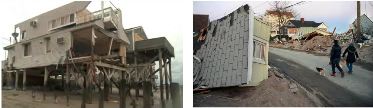
Figure 2-2 Damaged buildings on Fairfield Beach Road during Hurricane Sandy
