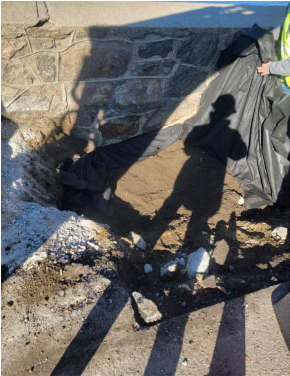
**Photo 4: Backfill of test pit with filter fabric, crushed stone, and excavated material**
